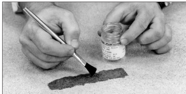
Figure 2 – Filling of the surface.
