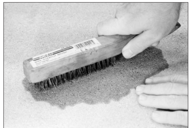
Figure 1 – Conditioning the surface for gage installation.
